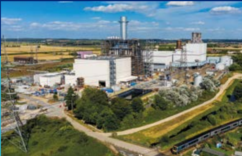
SSE is continuing to develop options for hydrogen blending technology at Keadby 2 in Lincolnshire
