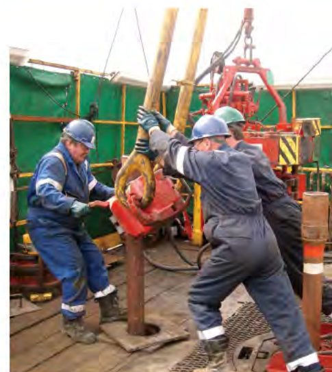
Construction work on Aldbrough Phase One
