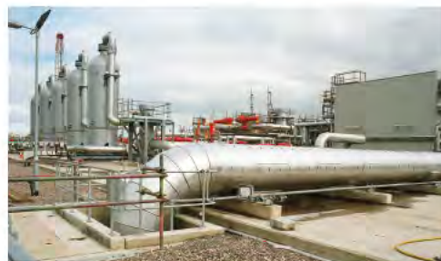
On site at Aldbrough Phase One
