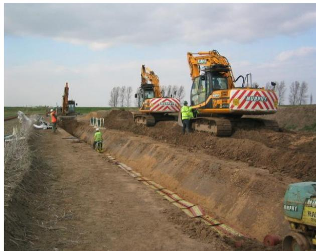
The maximum permanent cable route width required will be 13 m. For the majority of the route a maximum 30 m wide temporary working area will be required along the length of the cable route (known as the cable corridor). However, in some localised areas where HDD works are needed this corridor may increase to up to 40 m.
