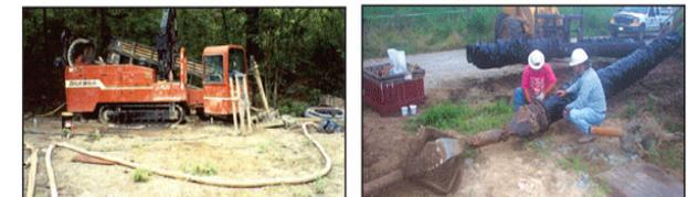
Cable installation onshore using directional drilling
