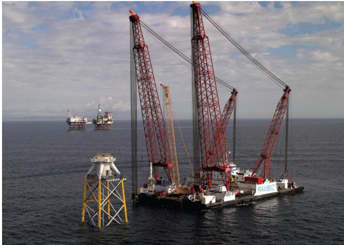
Typical construction vessel used to erect turbines
