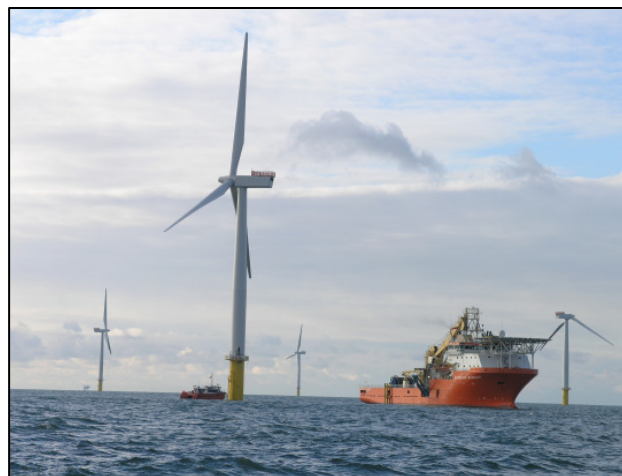
Wind turbine installation
