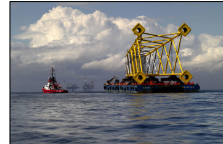
Substructure being towed to site
