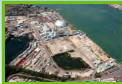
420MW of new CCGT capacity at Marchwood
