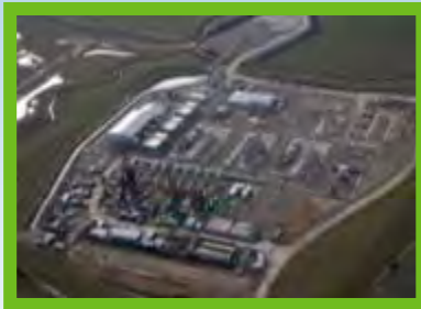
165mcm of gas storage capacity at Aldborough
