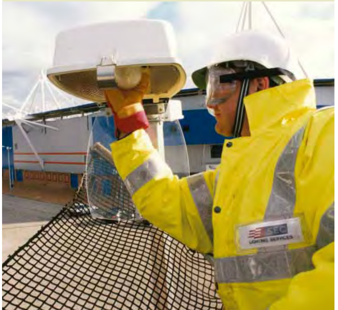
→ Right Contracting: SSE's Contracting Group maintains around one fifth of the street lights in England and Wales.
