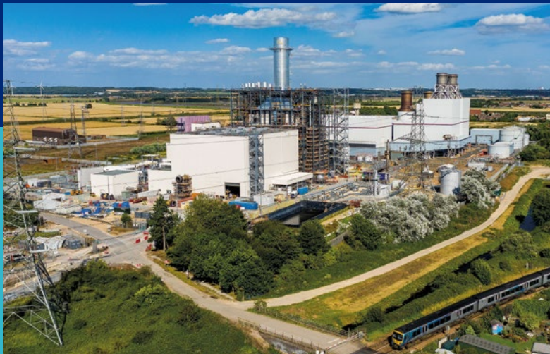
SSE is continuing to develop options for hydrogen blending technology at Keadby 2 in Lincolnshire
