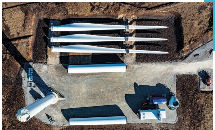
The component parts of one of the turbines at Viking wind farm
