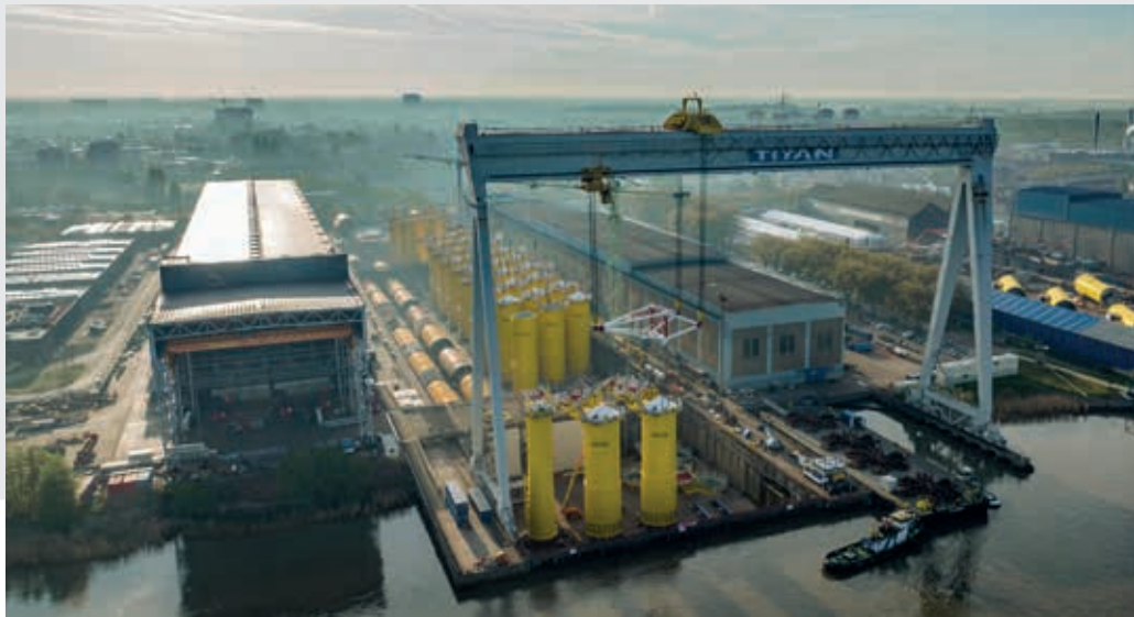
Turbine jackets ready for installation at Dogger Bank, the world’s biggest offshore wind farm.
